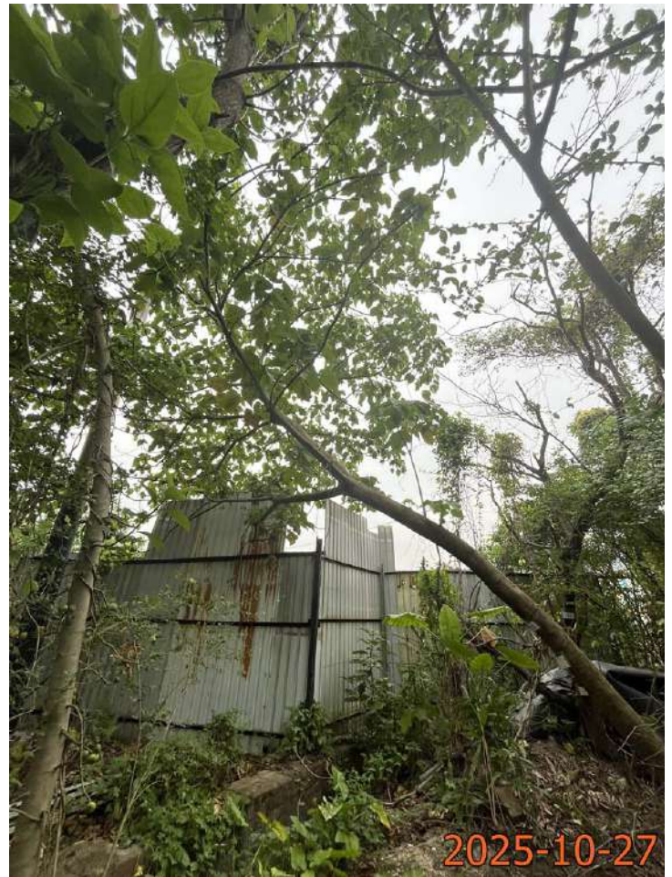
T23 (Overview) (Leaning)
